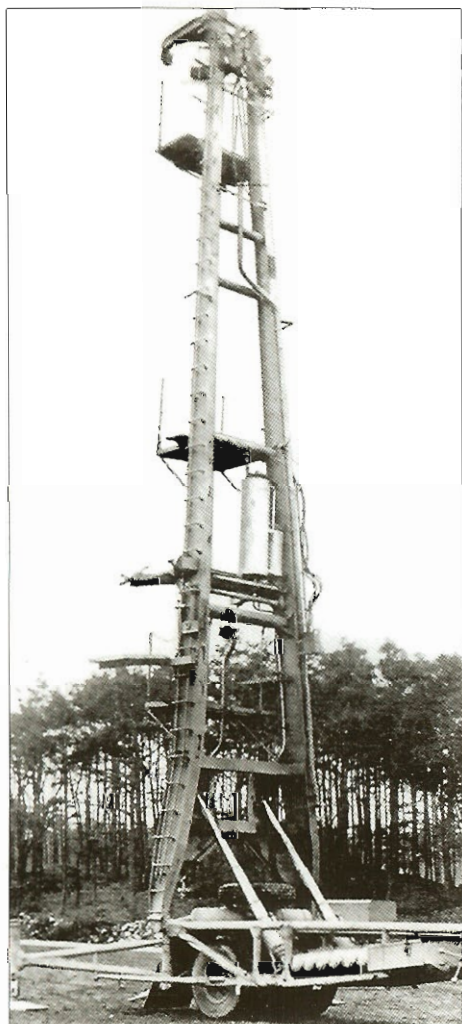
Left: The erected Starttisch (take-off table) with the hydraulic components and upper fold-out accessory platform.
