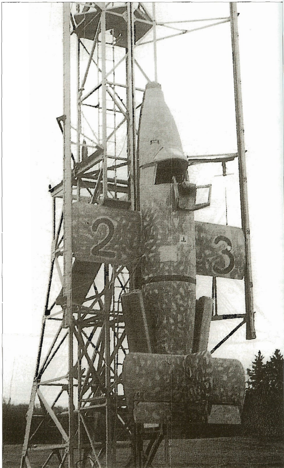
The Bachem BP 20 'Natter' M23 prototype with which Lothar Sieber undertook the world's first manned rocket-powered vertical take-off on 1st March 1945.
